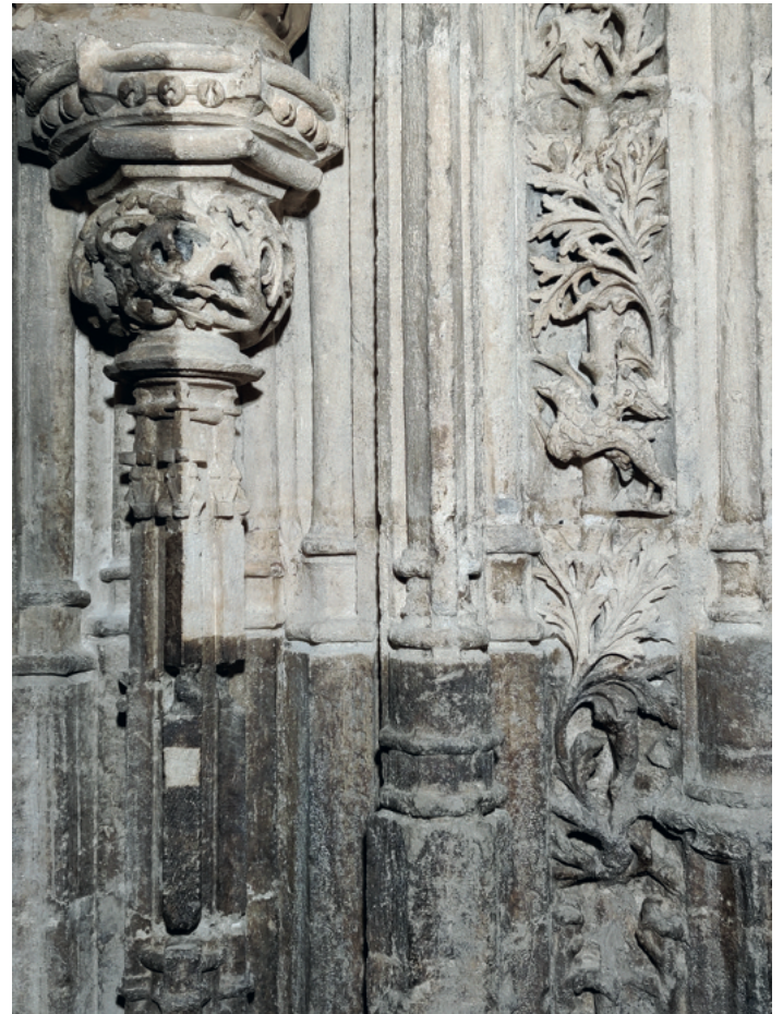
Fig. 3. Detail of the doorway during cleaning. ©Capilla Real de Granada
