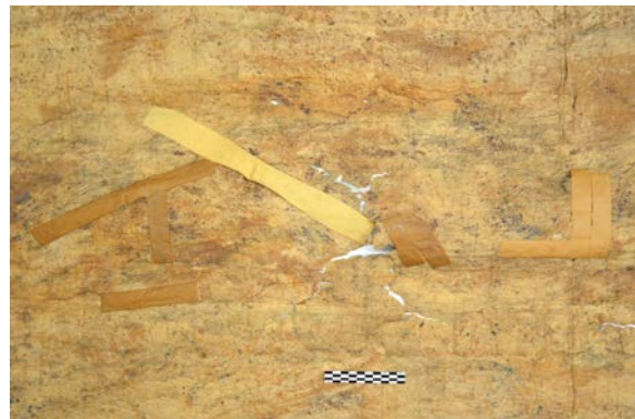
Figure 5. The three kinds of old repairs
