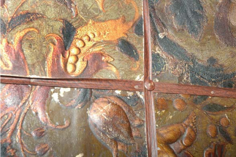
Fig. 1. The leather cloth strips covering the joins.
